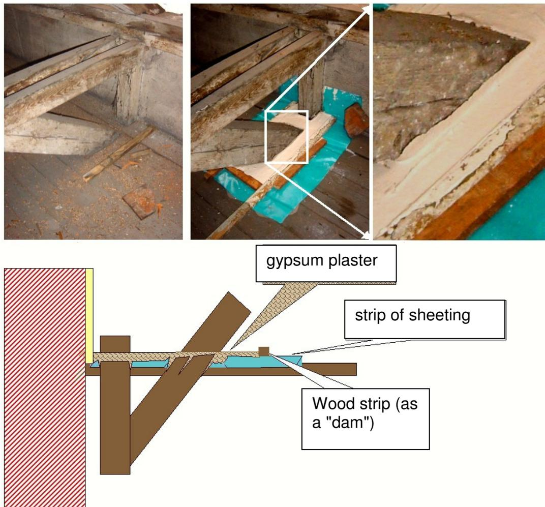
**Figure 29:** Poured gypsum plaster used in the refurbishment project Jean-Paul-Platz 4 in Nuremberg (Germany). Penetrating struts in the airtight layer of the top floor ceiling were sealed in this way (above left: initial situation with a strut; above centre: poured gypsum plaster; above right: detail showing the plaster which has poured into all cracks; below: schematic diagram (from [Feist 2003]).
