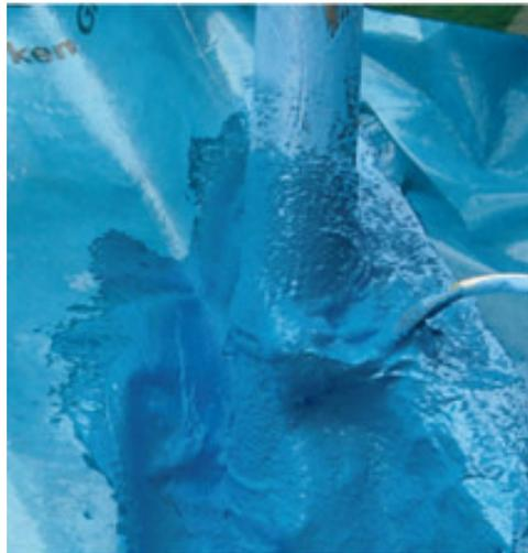
**Figure 14:** "Special solution" for sealing a penetration through sheeting, using a paste-like functional coating based on pure acrylate dispersion (source: Dörken GmbH & Co. KG)
