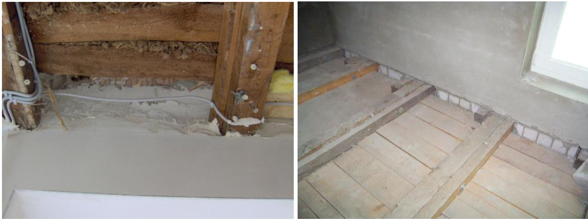
**Figure 7:** Partly exposed wood beam ceilings with wall supports of the wood beams in two refurbishment projects (Pictures: PHI)
