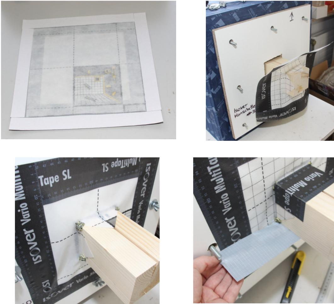
**Figure 27:** Pictures showing the work steps for a creating a sealing membrane collar (see text for explanations)
