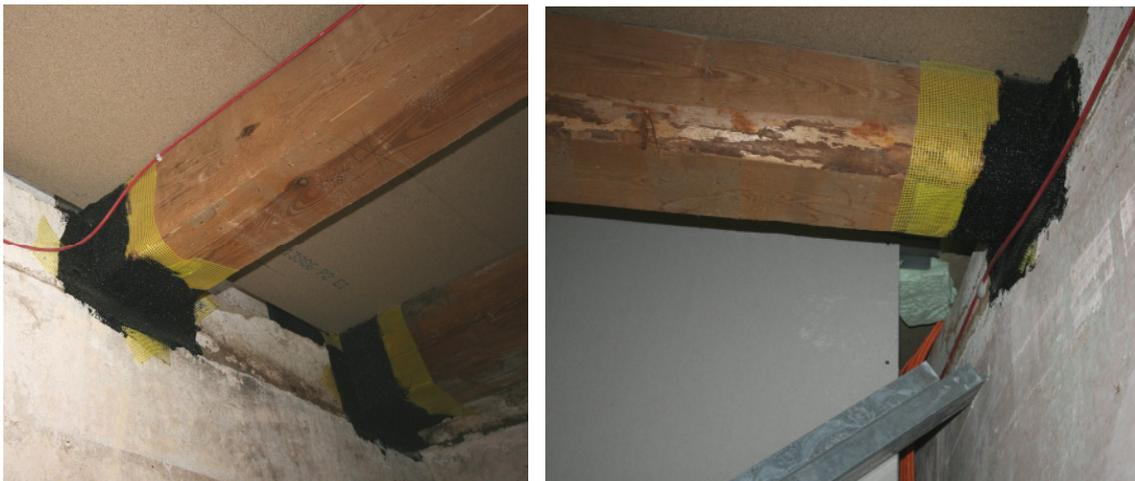
**Figure 31:** Example for the use of thick bituminous coating for sealing beams in the refurbishment project "Schloss Wartin" (Germany) [Hasper 2010]
