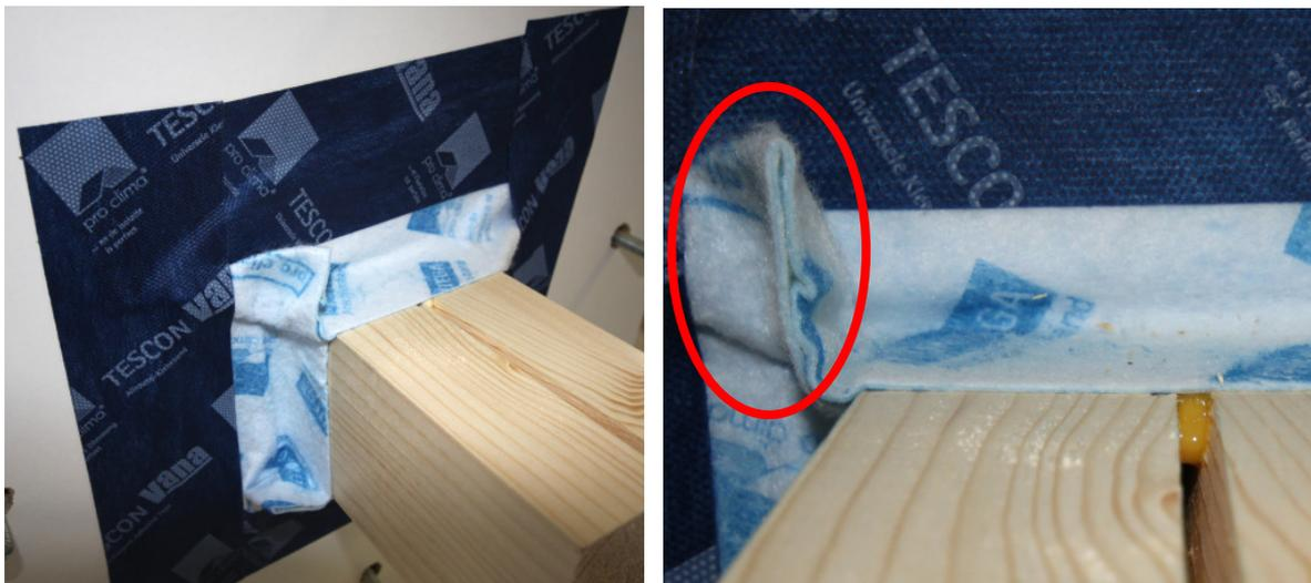
**Figure 23:** Beam sealed using plaster sealing tape (light blue) and joined to the cover using airtight adhesive tape (dark blue). In the detail on the right, a triangle formed with surplus sealing tape at the corner of the beam is shown (procedure in accordance with the manufacturer's instructions)
